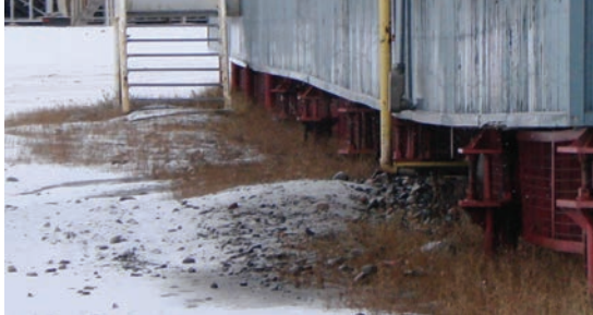
Uneven floors may indicate changing ground conditions.
