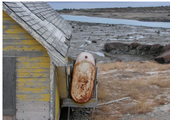
A wobbly or leaning tank can cause a break in your fuel line .
