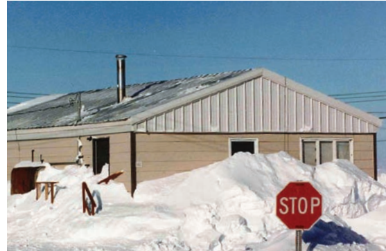
Snow banks insulate the ground, warming permafrost. Credit: RWDI Inc.
