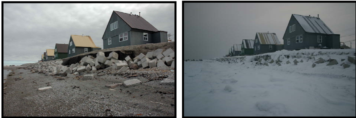
Figure 6: Summer (August) and winter (November) view of failed seawall.
