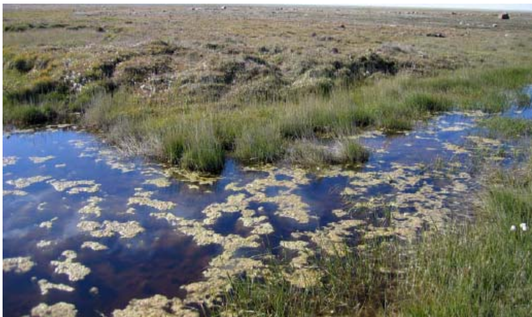
Figure 5. Thermokarst pond adjacent to the airport road, northeast of the runway. Construction of road blocked natural drainage allowing surface ponding of water which has thermally eroded ice-rich sediments below. Continued growth of the pond is seen by radially extending slump scars and collapse of 10 to 25 cm thick mats of peat into the pond, exposing underlying sediments to thaw and further settlement.
