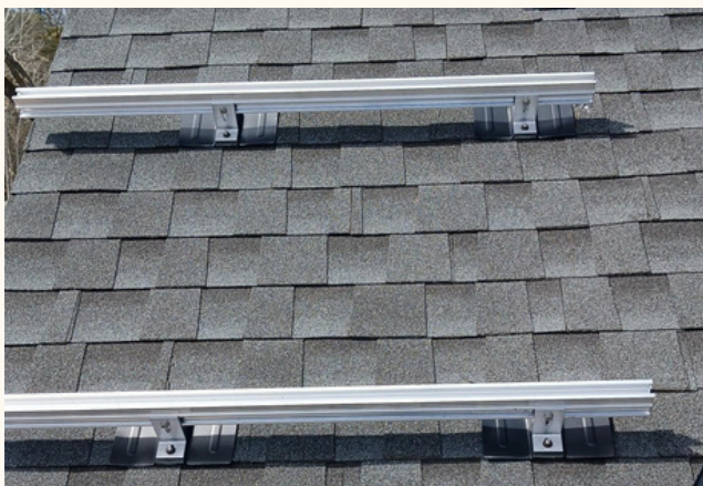
Rails mounted horizontally on a roof.
