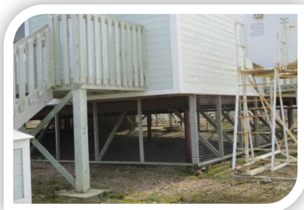
Examples of steel piles and mesh skirting around a house.
